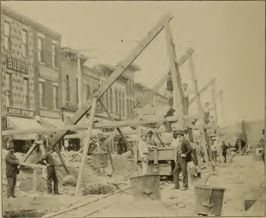
SEWER MACHINE AT WORK—AURORA, ILLINOIS.
